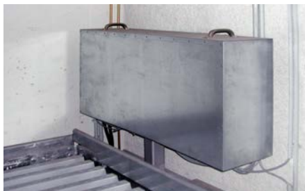
Sound insulation hood for the power unit
