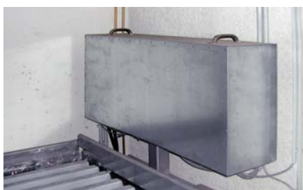
Sound insulation hood for the power unit
