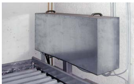
Sound insulation hood for the power unit
