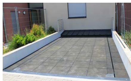
Rubber covering in stone structure (3 cm thick)
