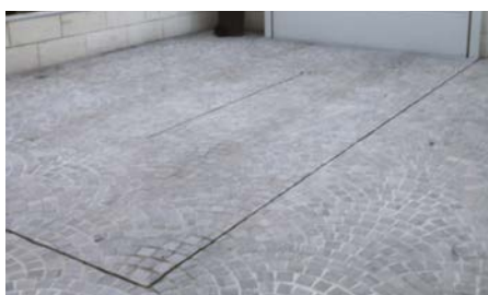
Synthetic stone covering (3 cm thick)
