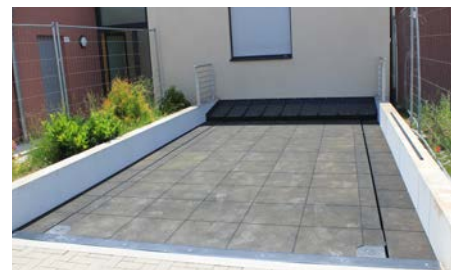
Rubber covering in stone structure (3 cm thick)
